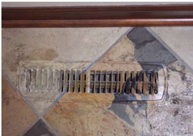
Clients often request Painting in Partnership to “make things disappear.” The craftsman used faux finishing techniques to complete this task.
